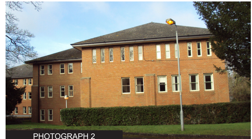
The rear (south) elevation of the late twentieth century office building.
