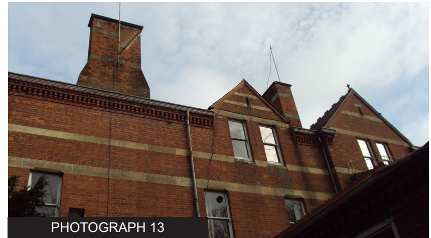
PHOTOGRAPH 13 The north elevation of Browfort
