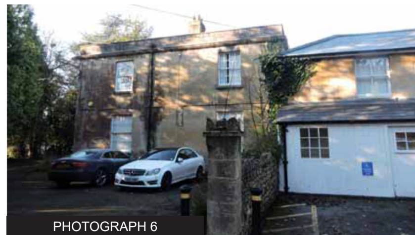
Rear of Cedar House from Dunkirk Hill side
