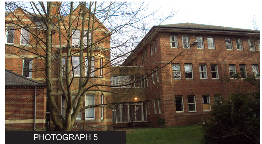
Rear (west) elevation showing link block between original 'Browfort' on LH side and modern office block to RH side
