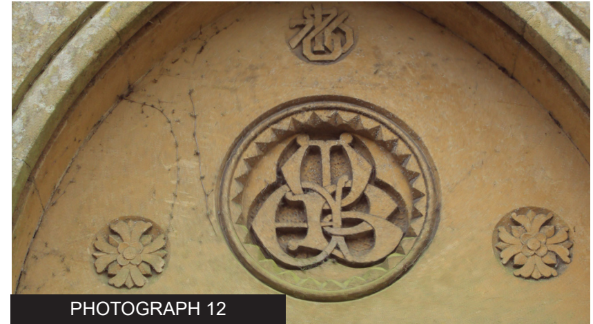
PHOTOGRAPH 12 The date of 1876 is just visible at the head of the recessed archway
