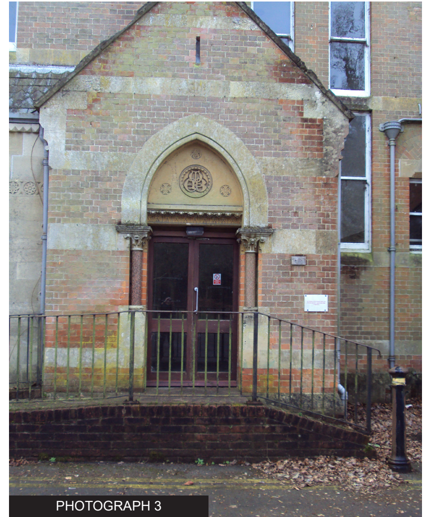
The original front entrance to 'Browfort' with raised ramp to left to provide disabled access.
