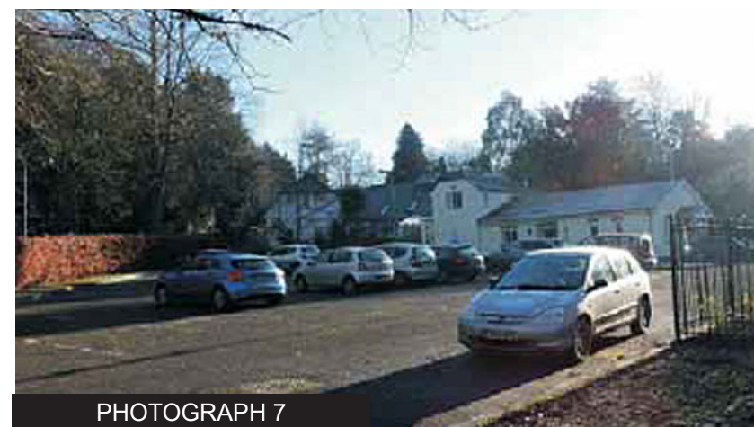
The former Browfort Lodge (RH middle ground) and the Cedars further to the left
