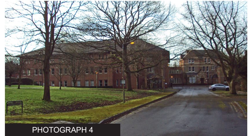
View westward from entrance drive with the 1876 'Browfort' to the right and the modern office block in the left foreground
