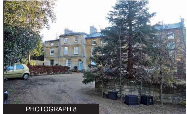
PHOTOGRAPH 8 Trafalgar Terrace - 1-5 Bath Road
